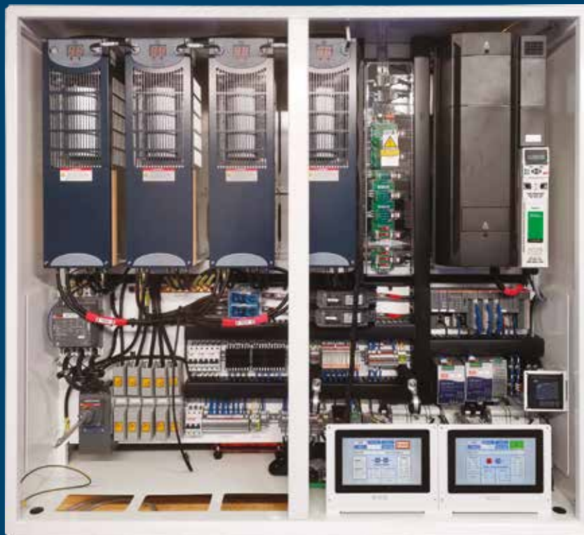
200 kVA Shore power combined 100kW shaft generator
