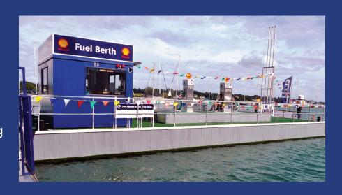
The structure is configured to provide buoyancy and to protect the fuel tank from damage. The unique design provides a safe, robust, stable and economic means of storing and dispensing fuel. The buoyant structure has a spillage containment area and a galvanized steel framework to receive the decking, fending and side skirts. It also incorporates the fuelling system and Kiosk control unit.
