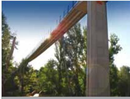
The world's longest stress ribbon bridge was awarded the JEC Innovation Award 2012 in the construction category. Future Fibres provided wound, unidirectional solid carbon fibre cables as the primary load-bearing supports of this footbridge built in Cuenca, Spain.
