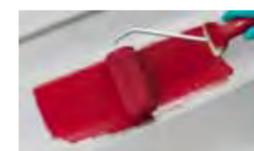
Avoid applying in adverse weather conditions, like strong wind, strong sunlight, high temperatures (especially at noon in summer time), low temperatures or high humidity or rain. It is not recommended to add solvents to antifoulings as this will reduce the thickness applied and increase the risk of sagging, splashes, etc.
