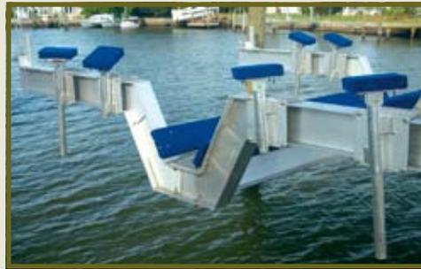
The 12,000 lb lift was specially built with a 24 degree angle to follow the slope of the rock wall. The heavy duty aluminum tracks were anchored to the rock face with large drilled anchors. This owner can now berth his boat in a location that was previously impossible.
