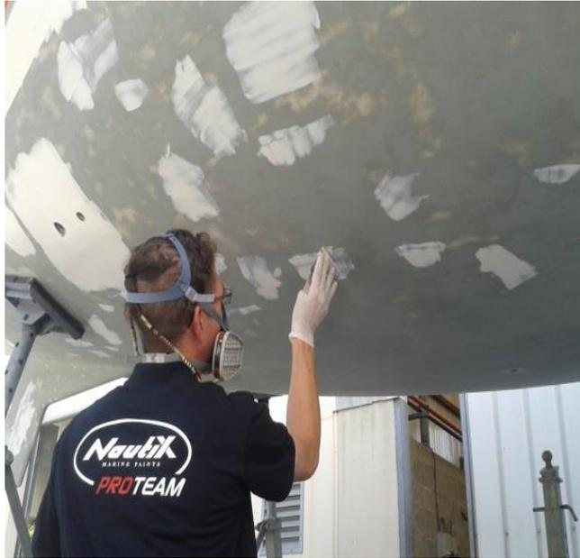
Fast-drying WATERTIGHT filler for low thickness application (5mm) and small local repairs (density 1)
