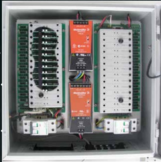
The brains in the system the type approved Lopolight Monitoring Relay
