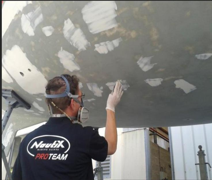
Application of filler is optional : depending on importance of surface imperfection (mixing ratio 1/1 in weight & volume)
