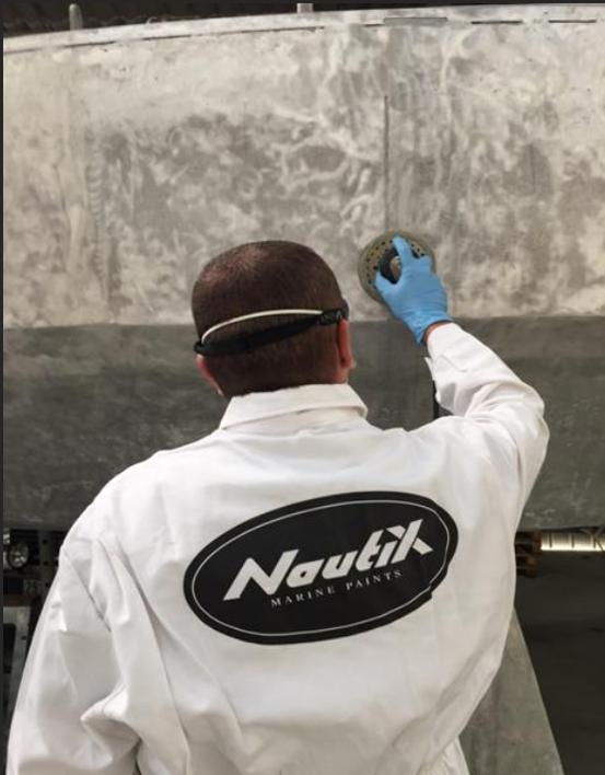
Clean the surface with soap, neutral or faintly caustic washing liquid (like diluted St Marc). Rinse with fresh water. If there is oil or fat, wash the surface with SD Nautix Degreaser.
