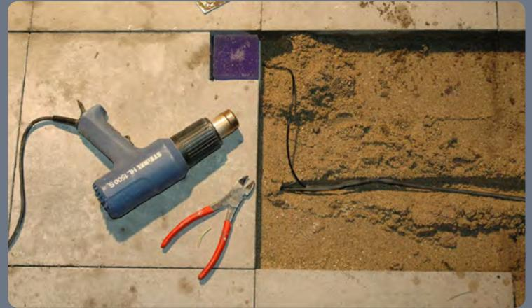
With a total depth of less than 3 inches Beckstone is ideal for renovation projects since it can be incorporated in the existing structure.
