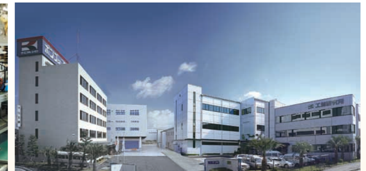
Head office and factory
