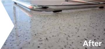
Concrete Terrazzo with the KGS RENOVATOR™ GREEN system (5 RENOVATOR™ + 3 FLEXIS® steps), average gloss level of 92% and a safe slip test result of 132.
