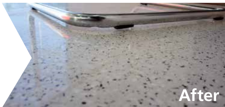
Terrazzo with the RENOVATOR™ STANDARD system, including the 4 RENOVATOR™ discs and the KGS polishing powder. Gloss level: 92%. Safe slip test result: 132.
