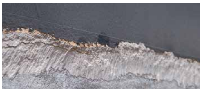
Removing thick layers of filler
